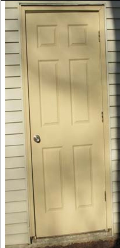
Six panel exterior grade doors are acceptable for outside closets. Match the style and color to rest of the building's rear closet doors.
